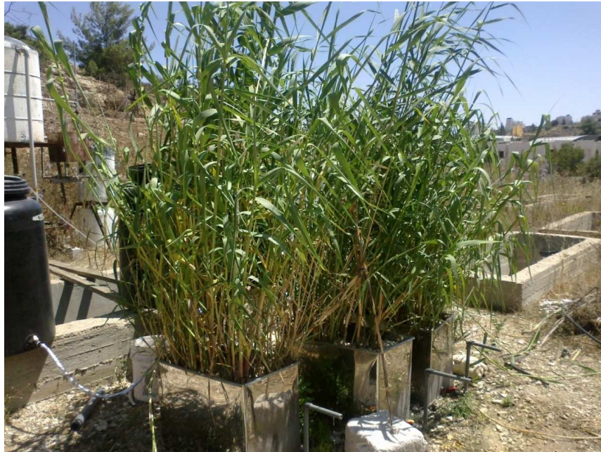
Photo 1 HSSFCW in operation, photo date (23/July, 2011)/ Birzeit University/ Palestine
